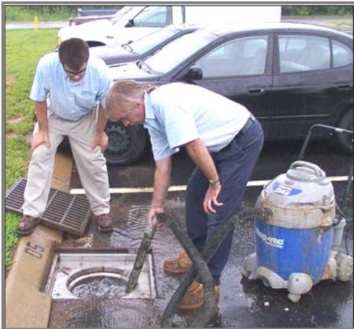
A shop vacuum cleans an Aqua-Guardian™ Catch Basin
